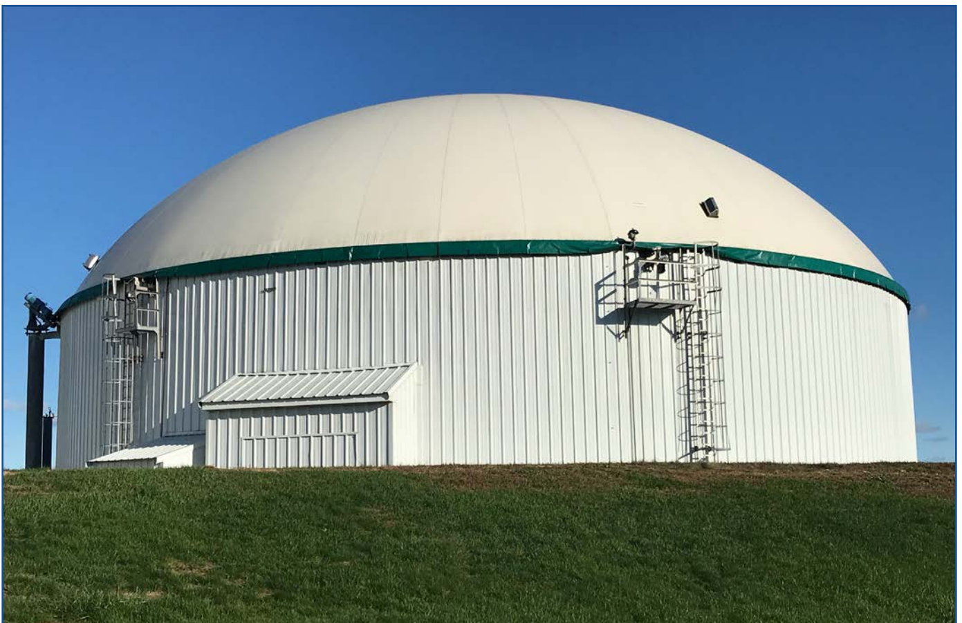
Photo 1: Dairy Biogas Anaerobic Digester Facility, Clean Fuel Partners, LLC, Dane, WI
