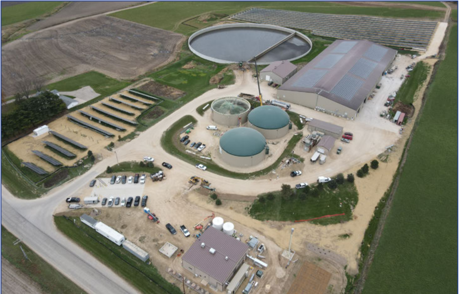
EnTech Solutions digester facility in Middleton, Wisconsin
