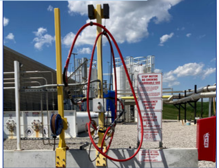
Top: Holding Tanks for RNG ready for transport, Left: Biogas digester digestate by-product for cow bedding, Right: Transfer station to load trucks for RNG transport to injection site
