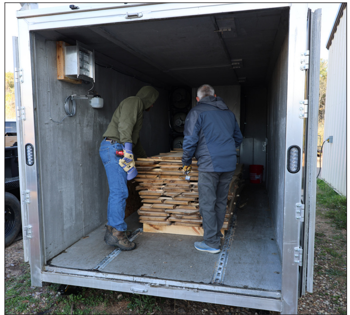
In August 2023 WFC staff, with guidance from Nyle Systems, finished constructing the first of two portable kilns. Built out of modified enclosed trailers and using Nyle Systems controls, the kilns will be used as part of the high school curriculum.
