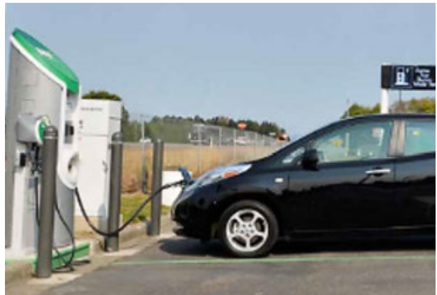
Figure 2.1. Level 2 chargers (top) are common in home, workplace, and public settings and can charge a BEV from empty in 4-10 hours. Direct-current fast chargers (DCFC) (bottom) are common as public chargers and along highway corridors, and can charge a BEV to 80 percent in under an hour. (Photos: ©123rf.com/ flippo [top]; Washington State Dept of Transportation [bottom])
