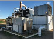
*Electrical generation from methane produced by digester*
