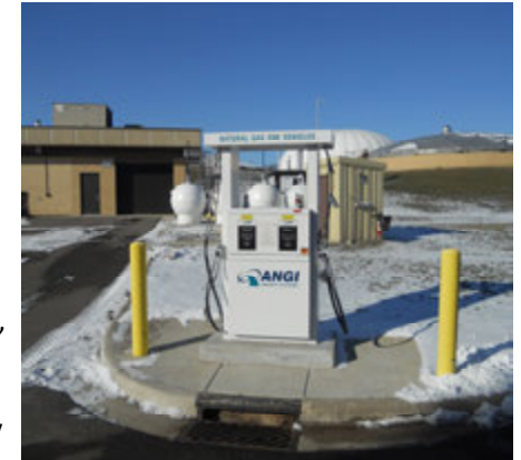
Photo B1: City of Janesville Fast Fill Gas Pump. The Janesville wastewater treatment plant produces biogas (bio-CNG) for use in municipal vehicles. (Photo courtesy of city of Janesville)
