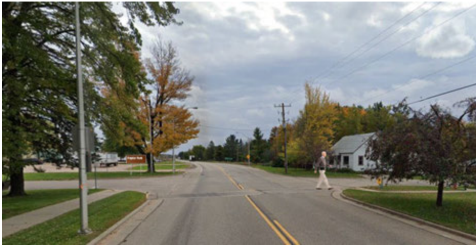
Crosswalk at the intersection of Highway 80 and poplar street
