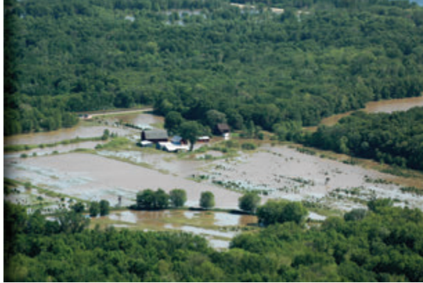
Figure T2 Flooded Farm, Rock County T4
