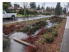
A rain garden alongside a road and sidewalk. It includes some native plants and grasses.
