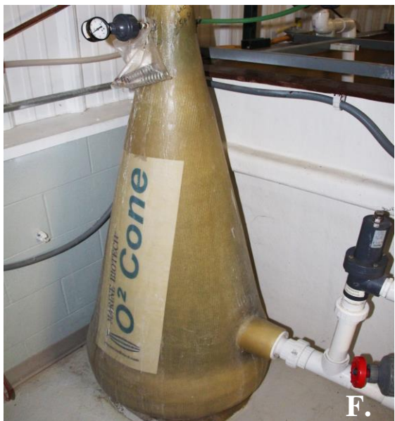
Fig. 50. Main Components of the RAS used to raise walleye at UWSP NADF. Culture Tanks (A.), Drum Filter (B.), Common Sump (C.), Fluidized Sand Biofilter (right in D.), Degassing column (left in D.), Ultraviolet Sterilization (E.), and Oxygen Cone (F.).
