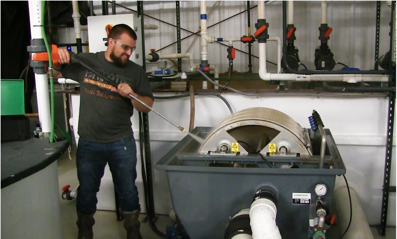
Fig. 62. Power washing drum filter as a regular maintenance of RAS.
