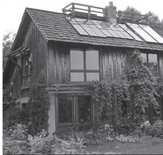
Photovoltaic panels mounted on the roof supply the household with electrical energy.
