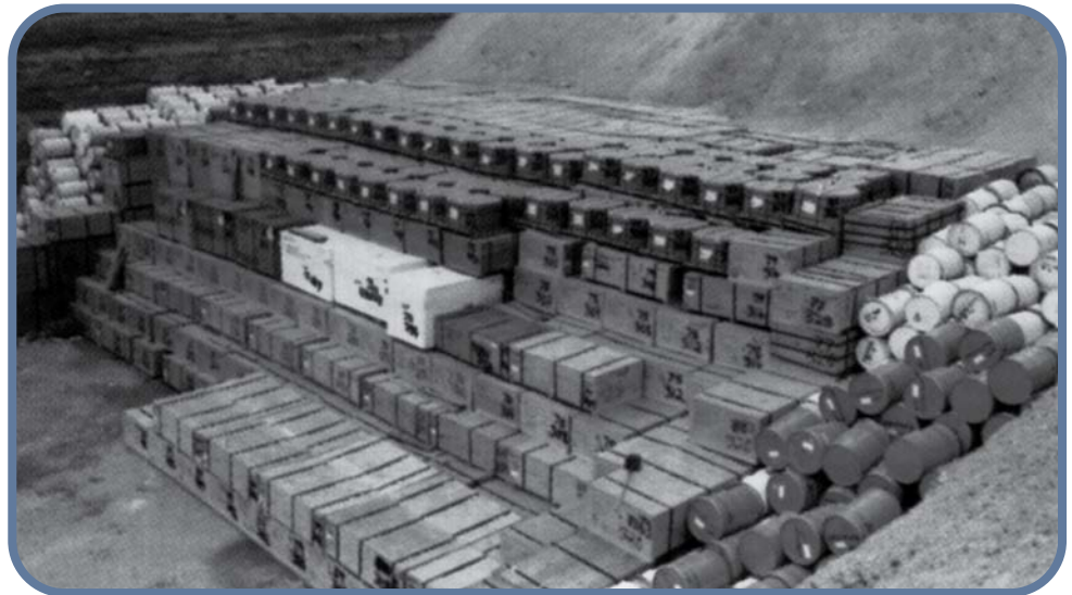
Solid low-level waste is safely disposed of in shallow trenches. When the trench is full, a protective covering for erosion control will be placed on top. Source: U.S. Department of Energy
