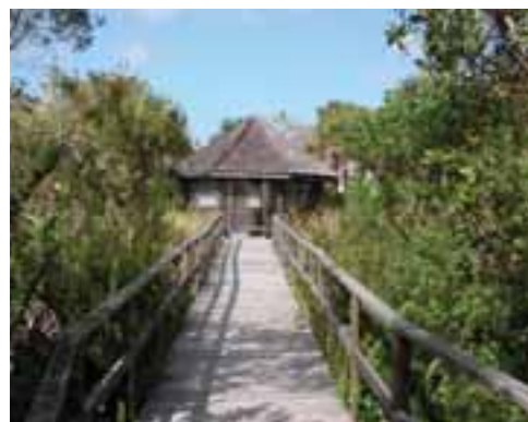
The boardwalk on the north part of segment 7 is accessible. The teaching shelter provides an introduction to ethnobotany.
