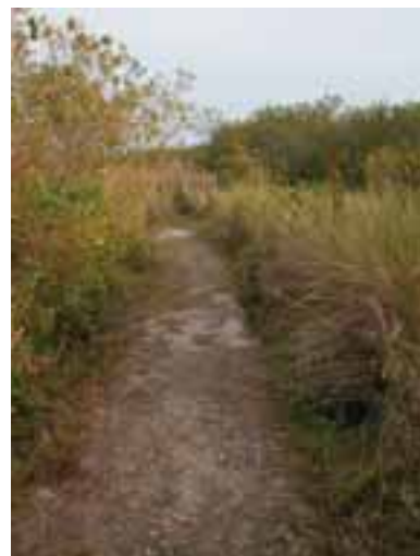
Segment 5 should be resurfaced with shell to provide better access.
