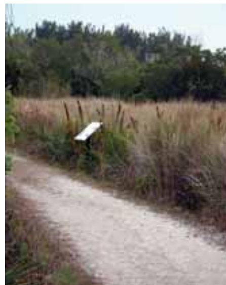
The south part of segment 7 should be resurfaced with shell to provide better access.
