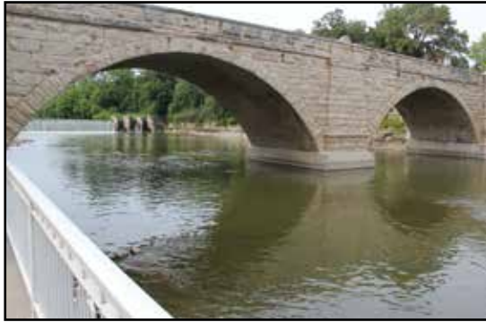
Keystone arch bridge in downtown Elkader
