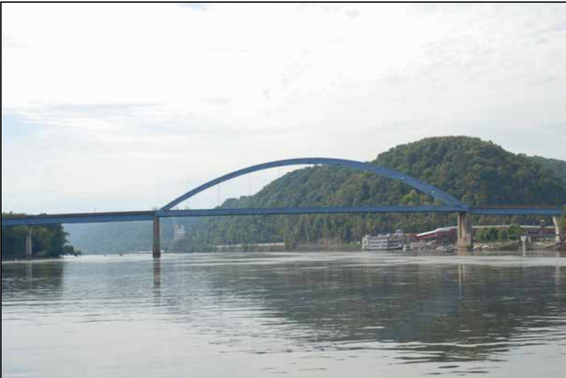
The Marquette-Joliet Bridge in Marquette connects Iowa with Prairie du Chien, Wisconsin.
