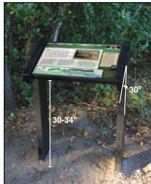
Aluminum frames and bases are attractive and durable. Setting the panel at recommended heights and angles ensures accessibility for the majority of visitors.
