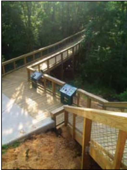
The boardwalk trail at Crowley's Ridge Nature Center in Arkansas protects the sensitive wetland habitat, avoids muddy ruts, and provides a solid walking surface for visitors.
