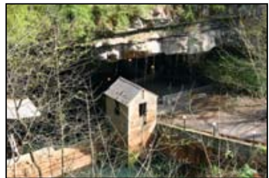
The dam and generator house were built in 1933 to supply electricity for the site.
