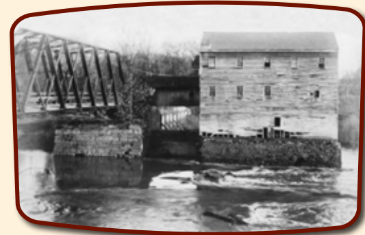
This photo shows the Old Iron Bridge spanning the Sangamon River next to the deteriorating Carpenter Mill, also known as the Rock Dam Mill. The bridge was dismantled in 1937 and set aside to be reused at another river crossing. However, it likely ended up as scrap for the World War II effort.
