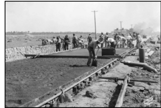
Laying brick road south of Springfield.
