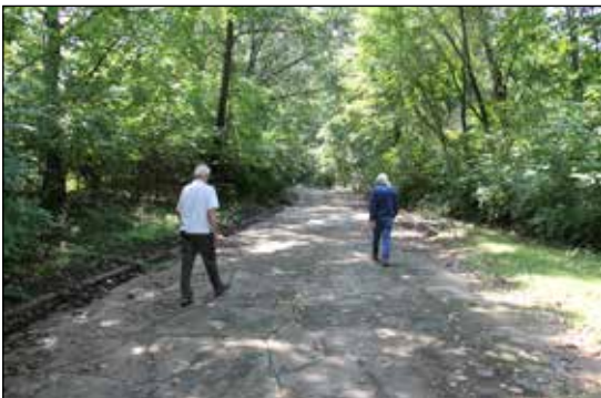
Carpenter Park Route 66 pavement (2021).
