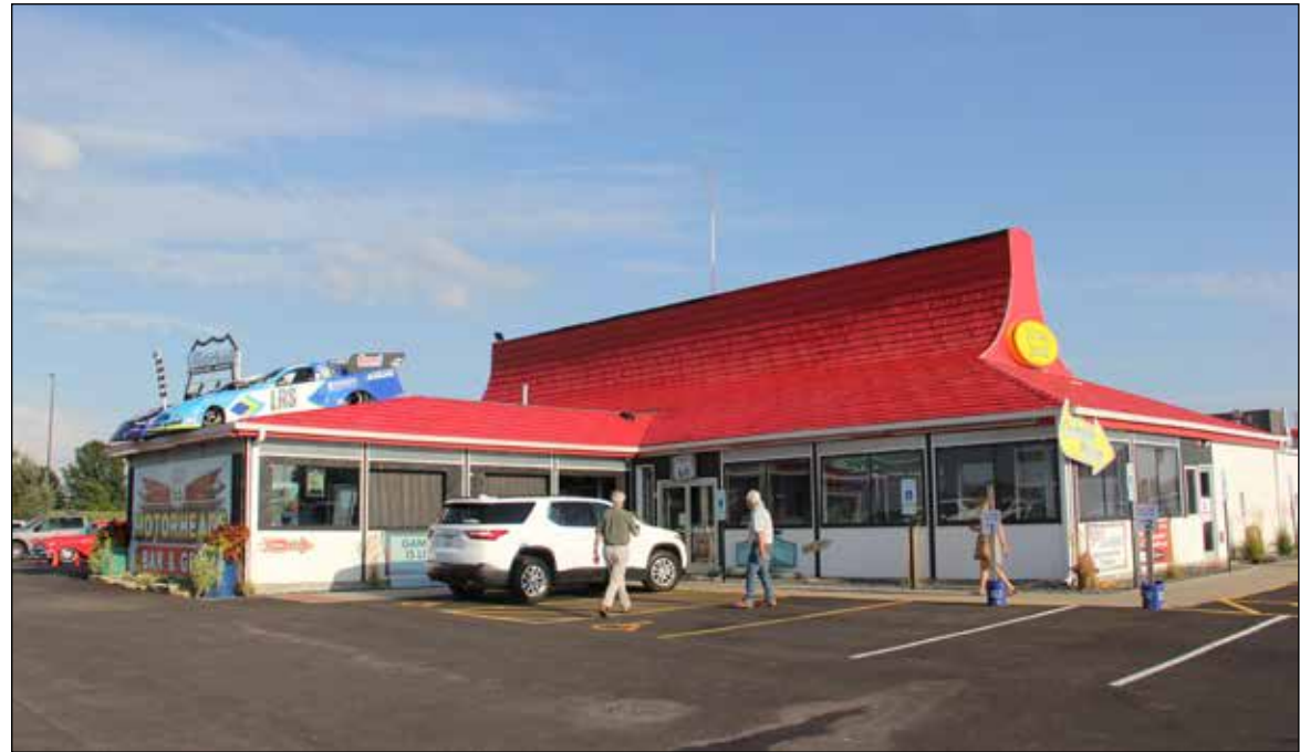
An experience hub should be located in a prominent location near the flow of traffic to be successful. Installing the hub near the entrance door of Motorheads would be ideal (2021).
