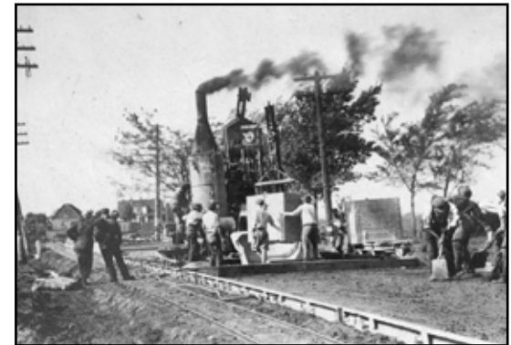
Constructing Illinois Route 4 near Springfield.
