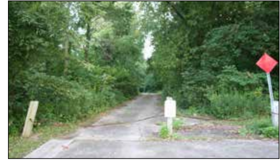
If the Carpenter Park pavement isn't developed as an interpretive trail, a wayside exhibit could be installed at the entrance (2007).
