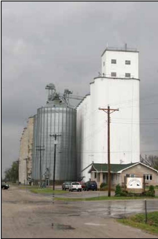
Grain elevators, like these near Elkhart, still dominate the landscape of rural Illinois communities along Route 66 (2007).
