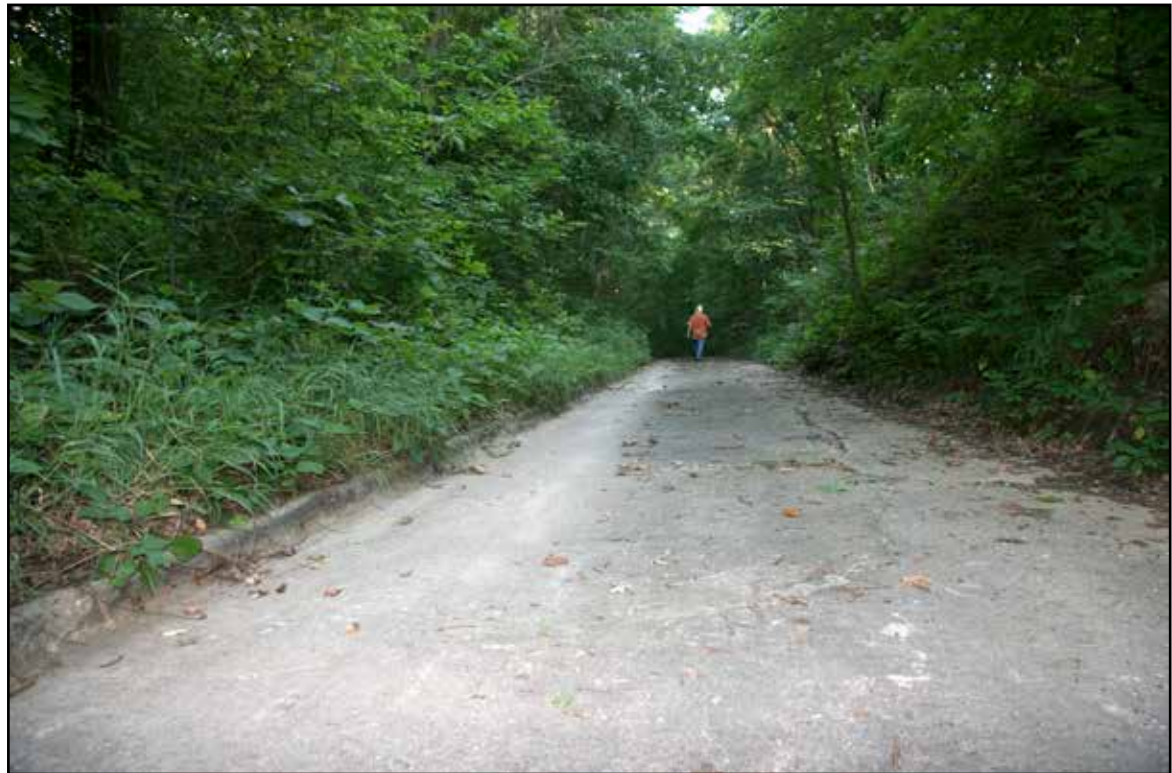
Original Route 66 pavement is still intact in Carpenter Park after it was bypassed in 1936 (2007).
