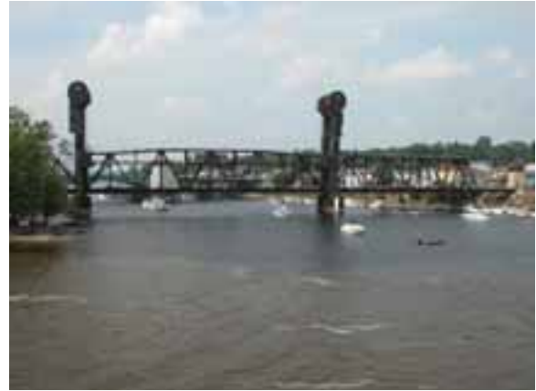
The Prescott railroad bridge spanning the St. Croix River.
