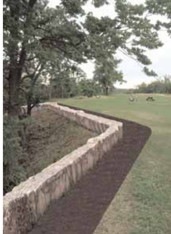
Limestone walls unify the bluff edge trail with other elements on the site, while a hard surface accommodates strollers and people in wheel chairs.
