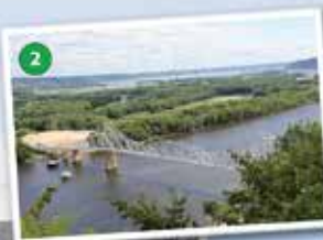
Black Hawk Bridge is an unusual steel truss bridge built in 1831.
