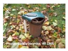
Cracked or poorly sealed well caps can provide insects and other organisms a pathway into your well.
