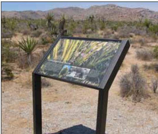
Wayside exhibit with high-pressure laminate panel and cantilevered aluminum supports.
