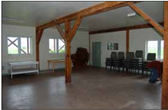
The finished space in the Slack Barn can serve education groups and visitors. The wood pillars somewhat reduce the flexibility. June 2011
