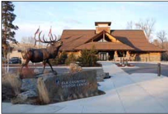
Elk Country Visitor Center, Rocky Mountain Elk Foundation. December 2009
