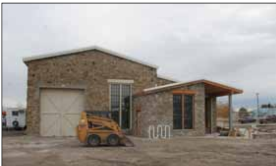
The Montana Outdoor Discovery Center under construction. October 2010
