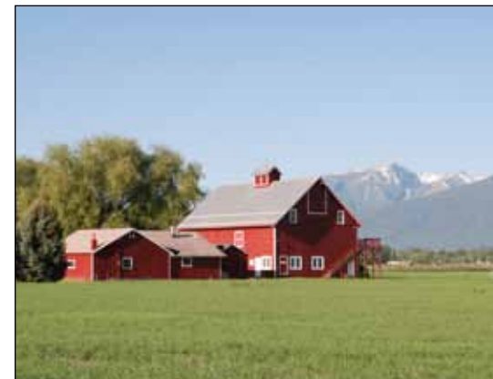
The Slack Barn serves as an important gathering place and adds to the classic ranch setting. June 2010
