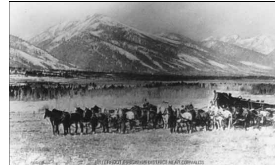
Excavating irrigation ditches near Corvallis.
