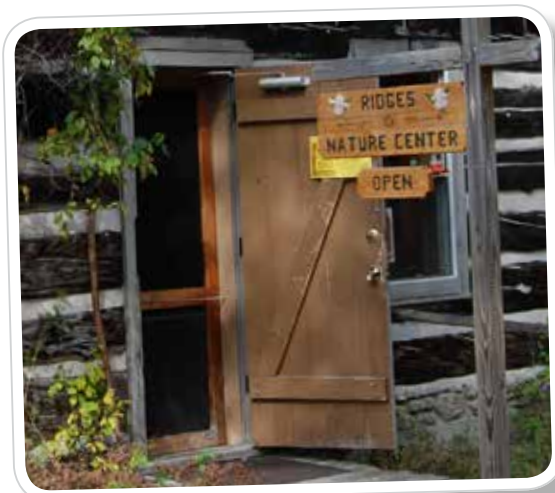
A screen door metaphor reflects the concept that the building is only a gateway to an outdoor experience.
