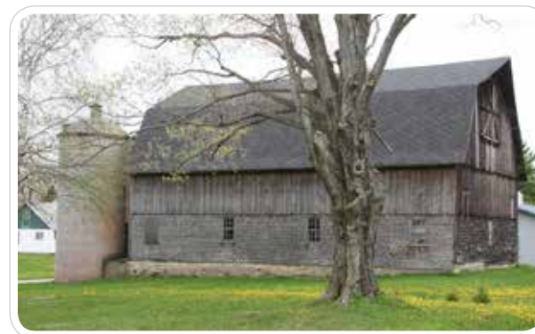
The vernacular architecture of the Peninsula includes limestone foundations and pine board siding.
