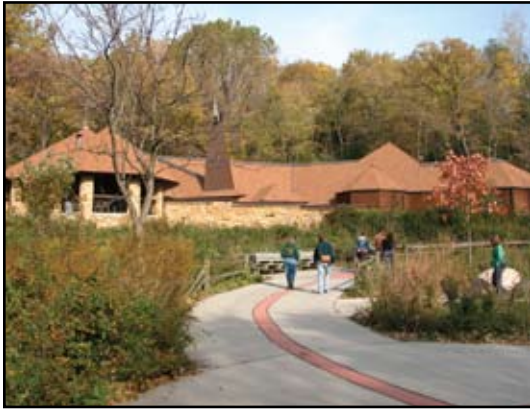
Guidelines for effective interpretive center design include respecting the landscape and culture of a region, reflecting the natural characteristics of a site, planning a color scheme that complements the landscape, and incorporating sustainable features. The Savage Visitor Center in St. Paul, Minnesota is built from the native limestone that surrounds the building.
