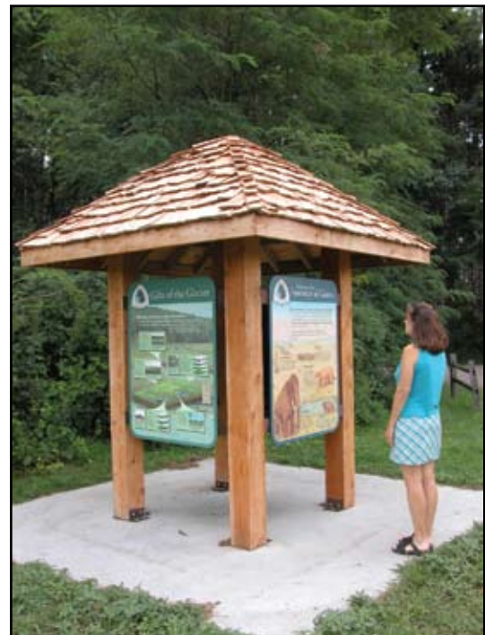
This roofed kiosk at Hartman Creek State Park interprets the Ice Age Trail in Wisconsin with dramatic visuals and a rustic design.
