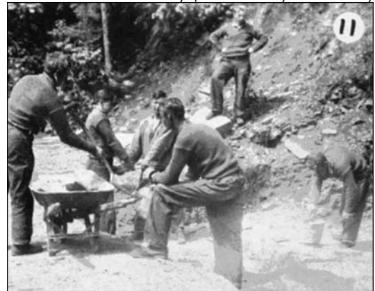
Members of the 3649th CCC camp worked on paths, roads, campgrounds, and buildings at Rib Mountain State Park.
