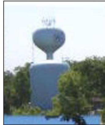
City of Waupaca water tower
