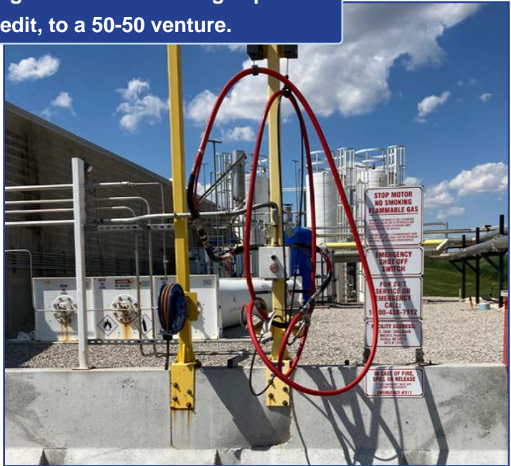
Top: Holding Tanks for RNG awaiting transport; Left: Biodigester digestate by-product for cow bedding; Right: Transfer station to load trucks for RNG transport to injection site
