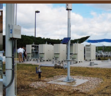
Microturbines at the Sauk County, Wisconsin, landfill.
