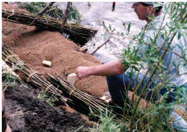
Erosion control fabric on a vegetated geogrid.
