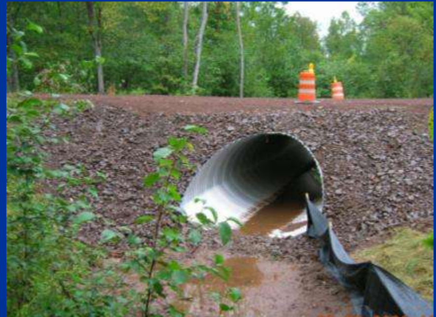
7' x 11' x 60' pipe arch culvert
