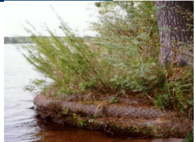
1-3 tiered with wood stakes
