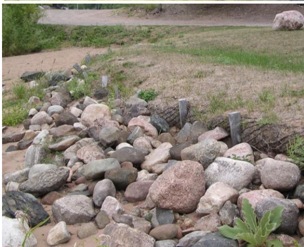
1-2 tiered with wood stakes & rock
