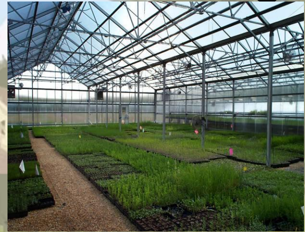
Taylor Creek Restoration Nursery Greenhouse; Brodhead, WI
