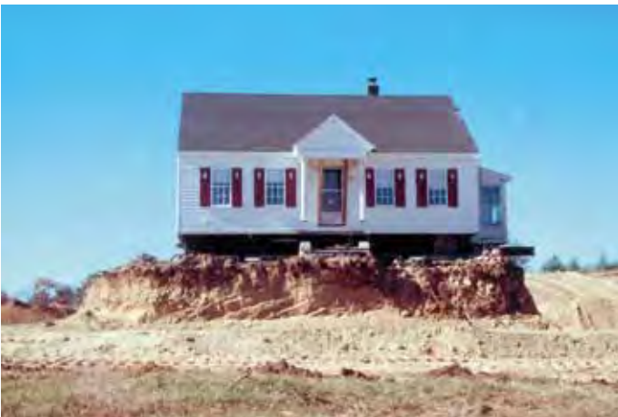
Low maintenance construction and landscaping is preferred to a no maintenance approach such as this.
