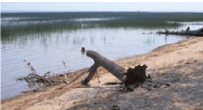
Pinconning outer bay, high water erosion in 1988.
