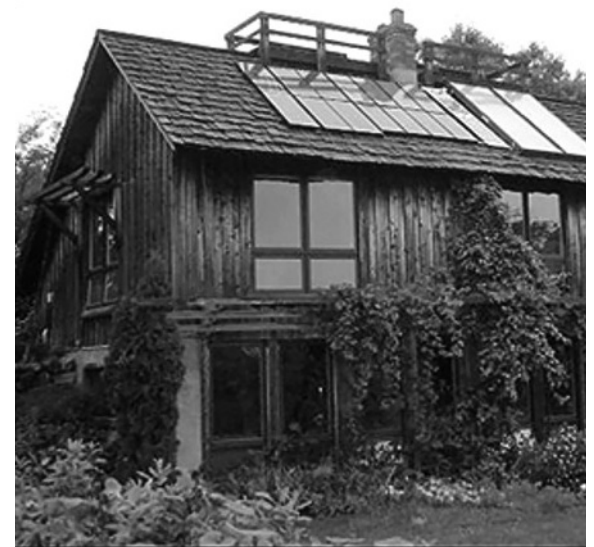
Photovoltaic panels mounted on the roof supply the household with electrical energy.
