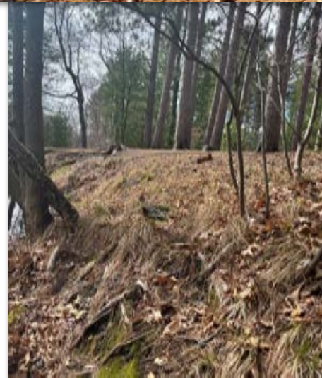
Figure 4: Image showing erosion in Little Plover Park along the Little Plover River.
