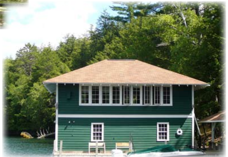
Boathouse classroom center
