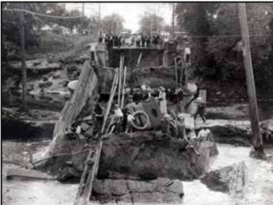
Squaw Creek bridge collapse in Ames, 1918
