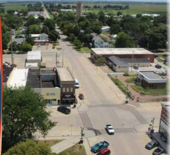
View of the Lincoln Highway heading east out of Jefferson from atop the Mahanay Memorial Carillon Tower
