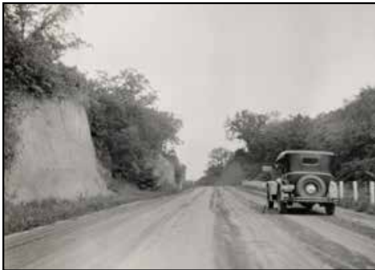
The Loess Hills created challenges for the early Lincoln Highway, requiring deep hill cuts, like this one at Honey Creek Hill north of Crescent.
