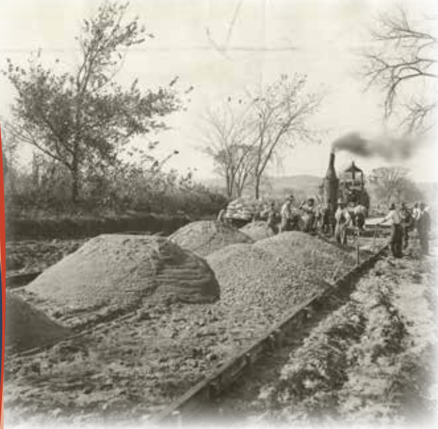
Concrete construction underway in central Iowa, 1915
