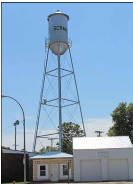
1897 Scranton Water Tower
