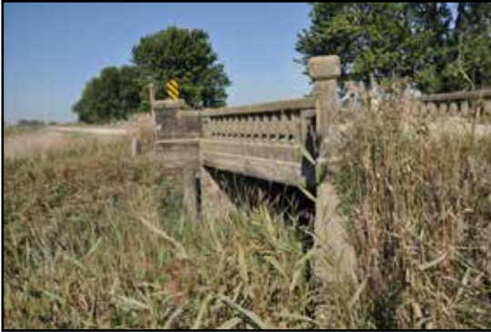
1915 "L" Bridge over Beaver Creek
