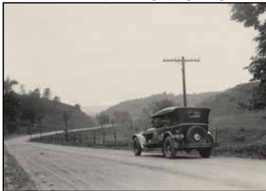
Lincoln Highway one mile west of Boone, 1926
