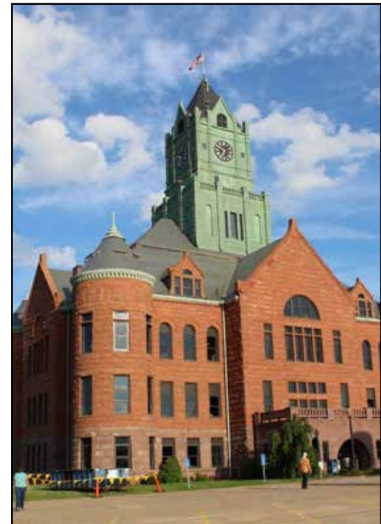
Clinton County Courthouse
