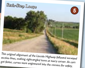
5 Snap-Step Loops This original alignment of the Lincoln Highway followed surveyed section lines, making right-angled turns at every corner. As cars got faster, curves were engineered into the corners for safety.
