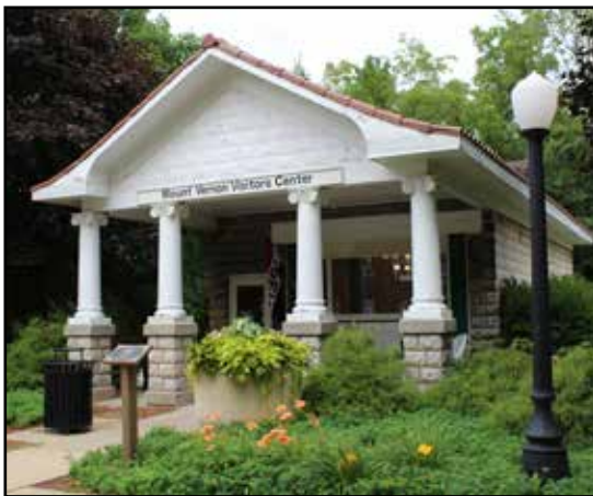
Mount Vernon-Lisbon Visitor Center in Memorial Park
