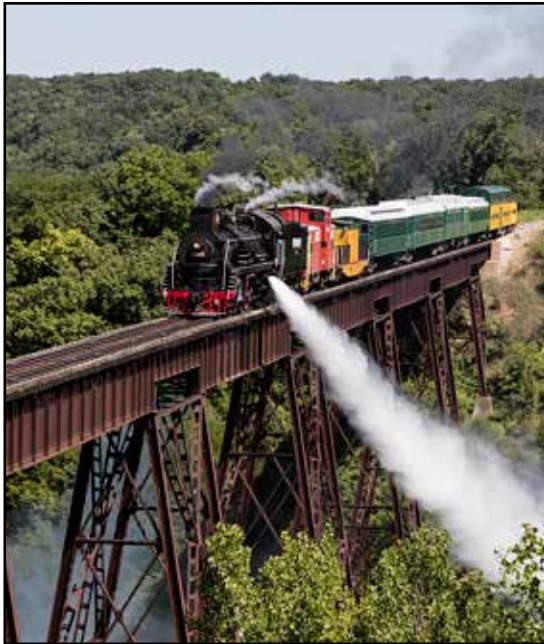
A Boone & Scenic Valley Railroad steam train crosses the Bass Point Creek Bridge.
