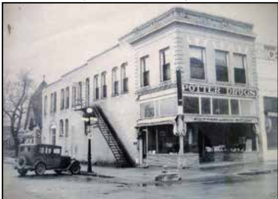
Historic Potter Drug Store building on the Lincoln Highway in Jefferson
