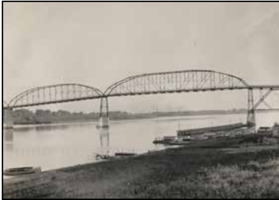
Old Fulton-Lyons Bridge, 1926
