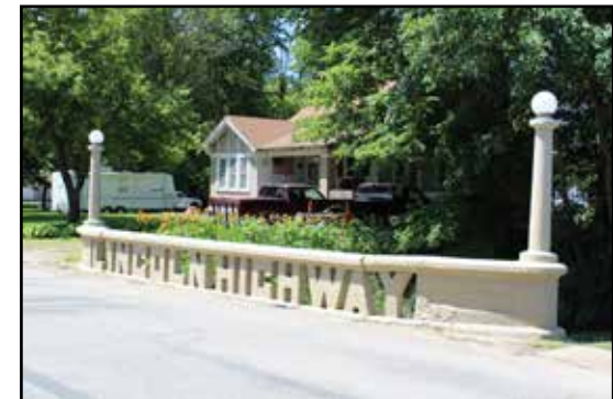
Lincoln Highway Bridge Park, Tama
