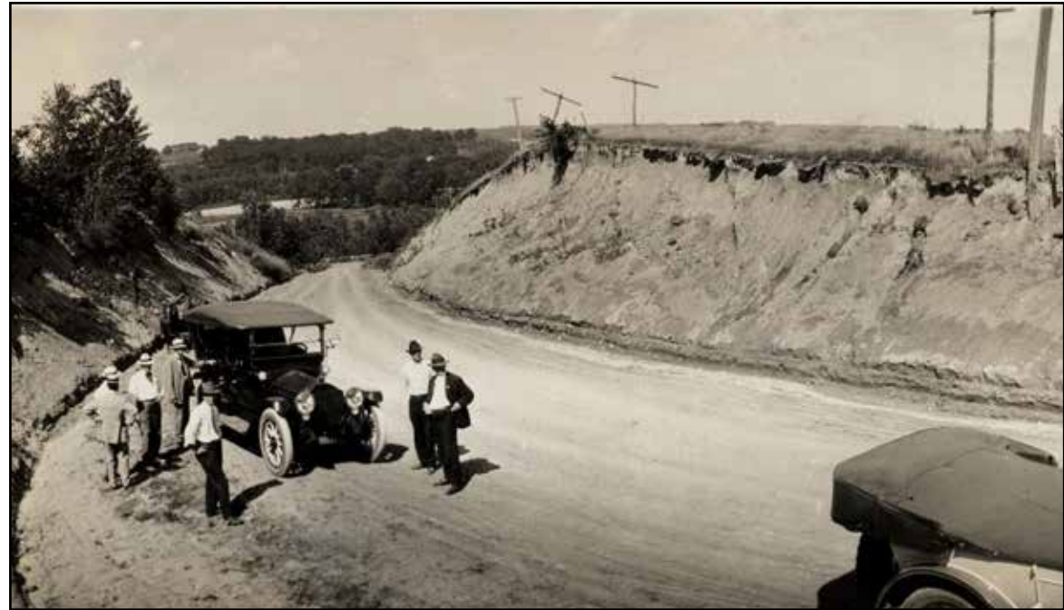
Heavy cut work and grading reduced the slope of Danger Hill west of Jefferson, 1918
