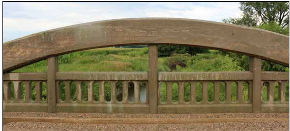
Marsh Rainbow Arch Bridge north of Beaver, Boone County
