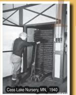
Cones on screen trays were heated in a *forcedair kiln* for 8 to 16 hours to open their scales.
