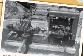
Two diesel powered pumps were installed first in 1931, and then the walls and roof were built around them. Later, they were replaced by electric pumps.
