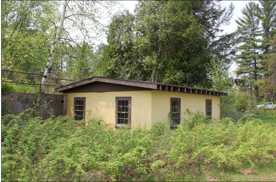
Figure 80. —Remaining lower floor of the Hugo Sauer Nursery seed extractory (map area #4) facing southwest, 2019.
