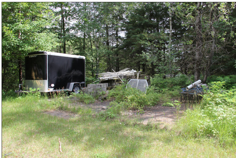
Figure 103. —The concrete slab at the south end of the loop drive in 2019 is where the Hugo Sauer Nursery Civilian Conservation Corps side camp kitchen building once stood (map area #12). A long mess hall oriented east-west stood in front of the kitchen.
