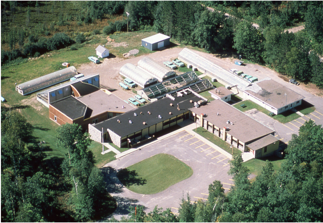
Figure 54. —The Forestry Sciences Laboratory in 1980 showing the 1972 wing addition (center with black roof) and the 1975 headhouse/greenhouse addition behind. USDA Forest Service photo archives.
