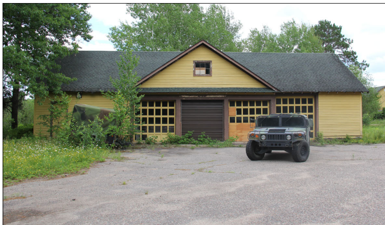
Figure 113. —Hugo Sauer Nursery repair shop (map area #17) facing southeast, 2019.
