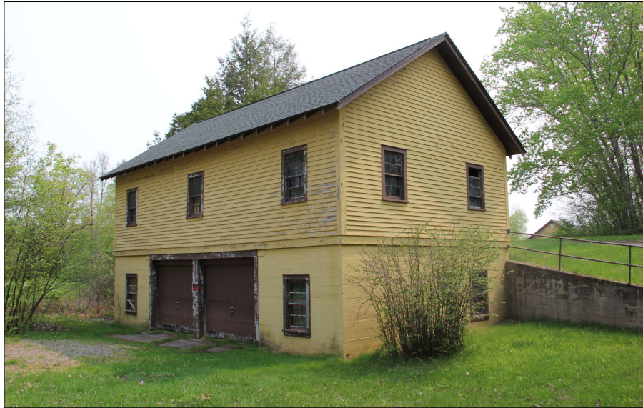
Figure 82. —Both stories of the Hugo Sauer Nursery warehouse #1 (map area #5) facing northeast, 2019.
