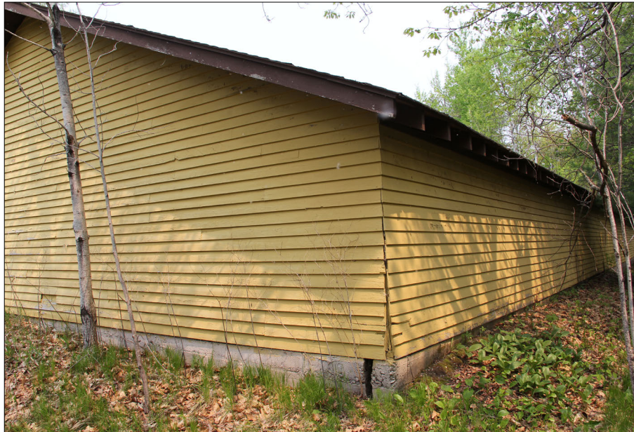
Figure 100. —Hugo Sauer Nursery implement shed backside (map area #11) facing north, 2019.
