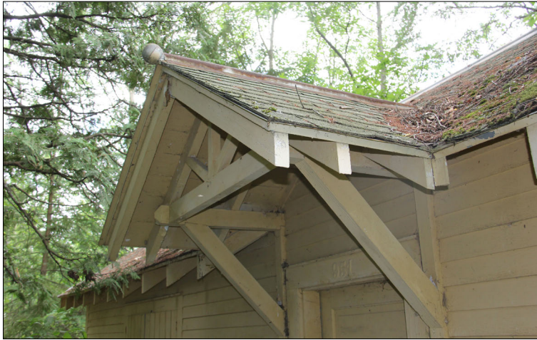
Figure 108. — Gabled roof and decorative features over the front door on the east side of the Hugo Sauer Nursery pumphouse #2 (map area #14), 2019.
