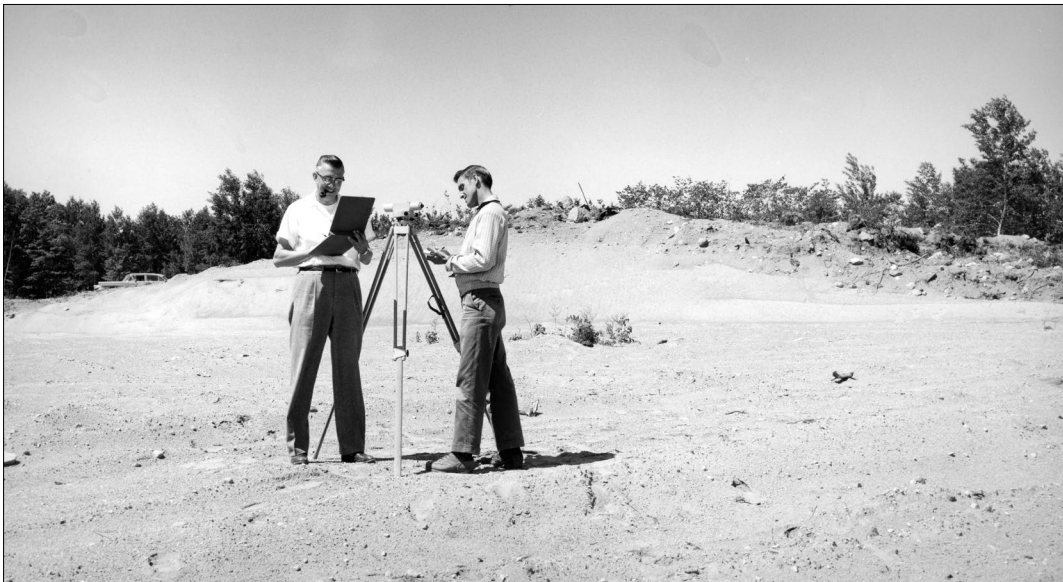
Figure 47. —Hal Luedtke (left), administrative assistant, and Art Flancher (right), engineer, establish final grade for the original radiation field at the Institute of Forest Genetics in 1964. USDA Forest Service photo archives.
