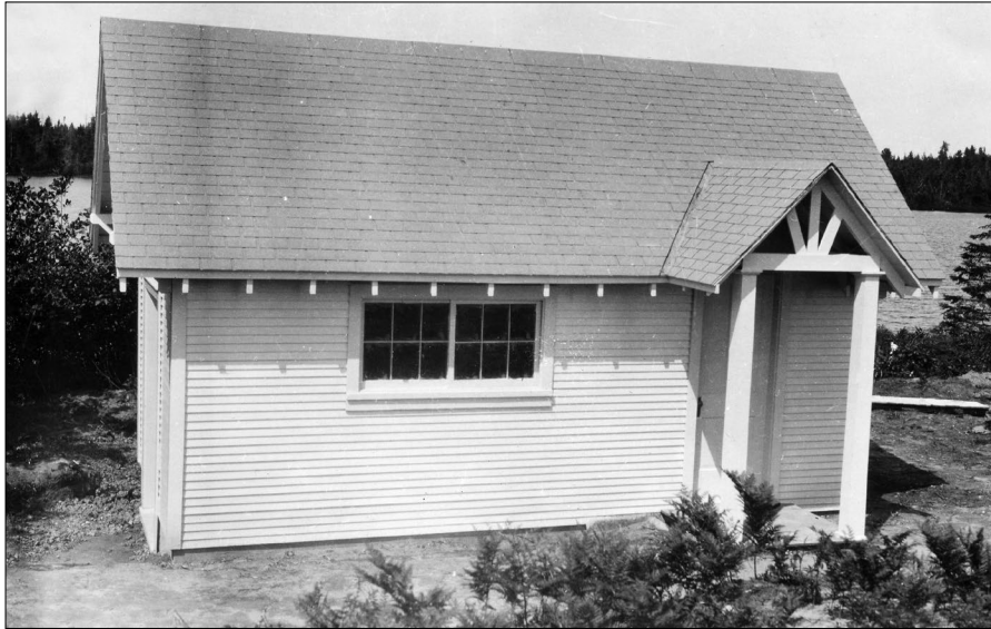
Figure 89. —Hugo Sauer Nursery pumphouse #1 (map area #8) facing west, 1931. USDA Forest Service photo archives.
