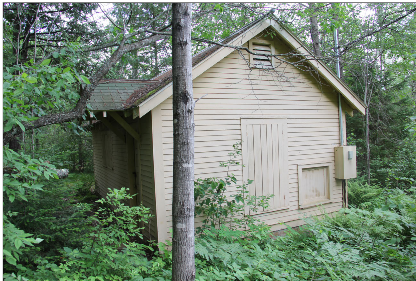
Figure 107. —Hugo Sauer Nursery pumphouse #2 (map area #14) facing southwest, 2019.
