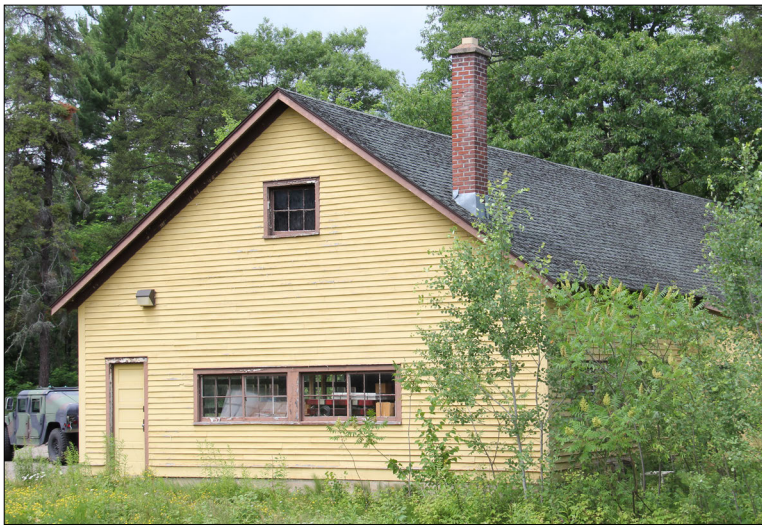
Figure 115. —Hugo Sauer Nursery repair shop (map area #17) facing northwest 2019.
