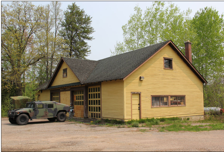
Figure 114. —Hugo Sauer Nursery repair shop (map area #17) facing north, 2019.
