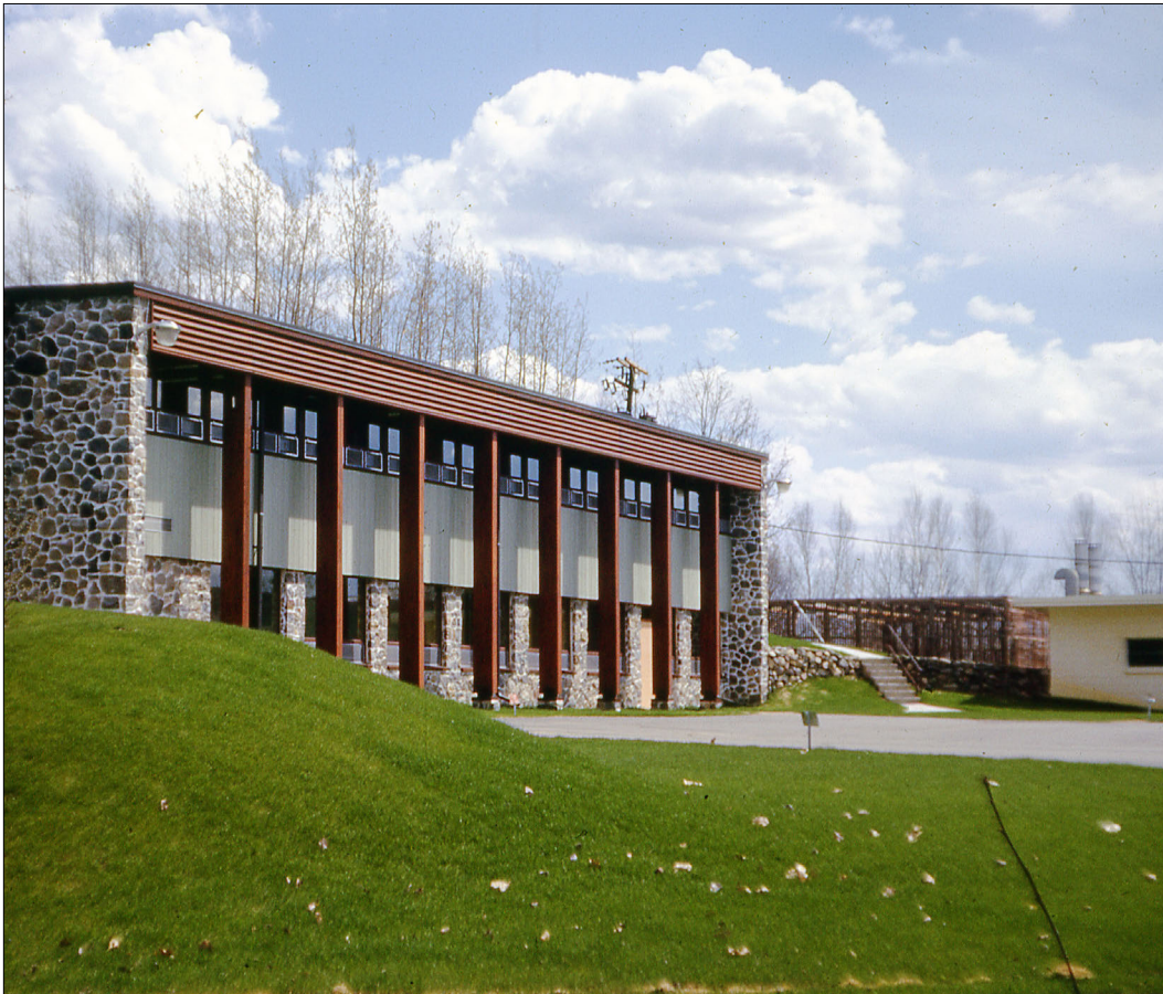
Figure 39. —A southeast view of the newly constructed Institute of Forest Genetics building in 1962, showing both stories exposed with exterior stonework and laminated columns. USDA Forest Service photo archives.
