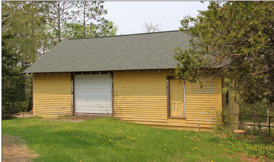
Figure 83. —Top story of the Hugo Sauer Nursery warehouse #1 (map area #5) facing west, 2019.
