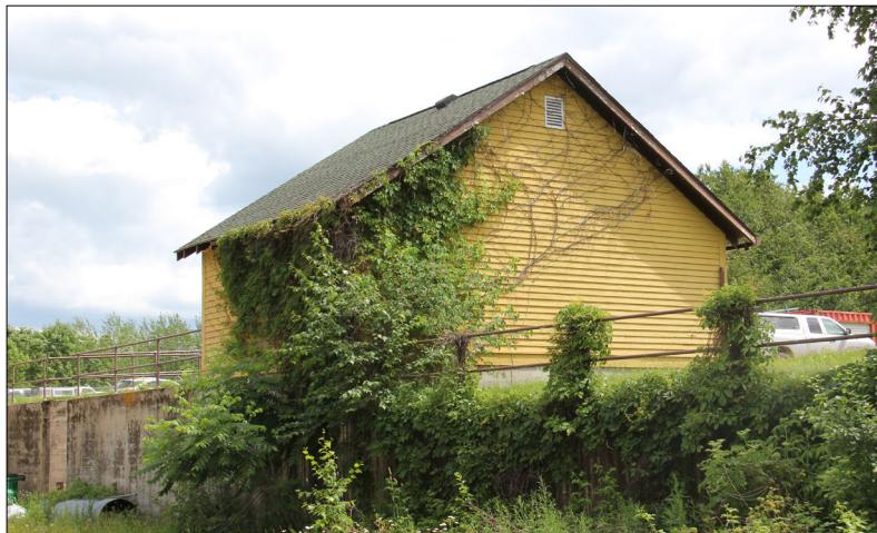
Figure 86. —Hugo Sauer Nursery seed storage shed (map area #6) from the bottom of the retaining wall facing southeast, 2019.
