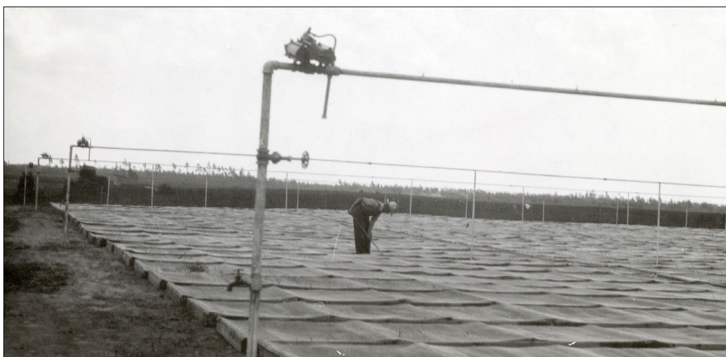
Figure 22. —The Rhinelander nursery's overhead irrigation system as it appeared when installed in 1931. The vertical pipe risers connect the overhead sprinkler pipes with the underground water pipes. The wire screen over the beds protects the seedlings from birds and rodents. USDA photo archives.
