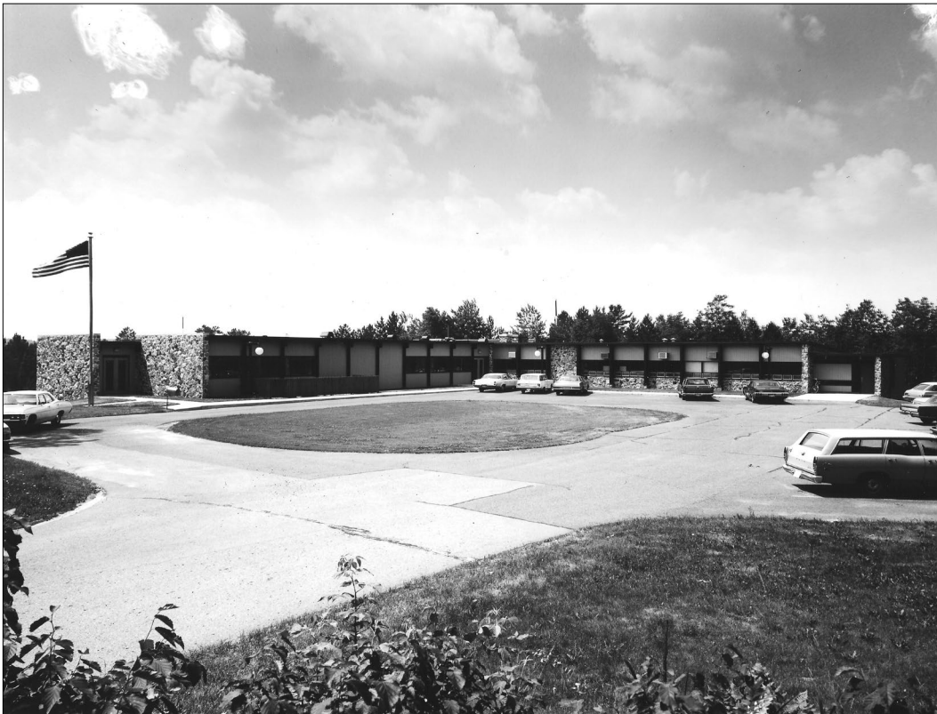
Figure 53. —The Forestry Sciences Laboratory in the mid-1970s showing the 1972 wing addition (left) attached to the original building (right). USDA Forest Service photo archives.
