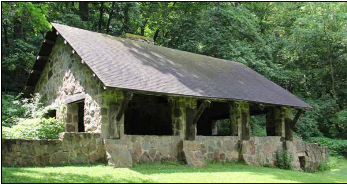
A Civilian Conservation Corps crew constructed the Wanata State Park shelter in 1934.
